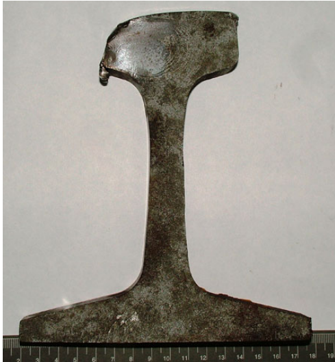
Figure 12: Broken rail due to Detail Fracture (TD) Defect
