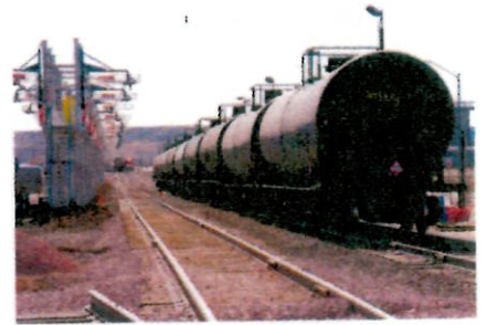
Great Western Railway serves this oil terminal at Windsor, Colo., which in November 2013 was building a two-track platform (left) to load unit trains. Chip Sherman
